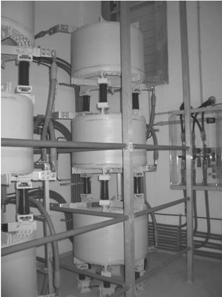
Figure 13.8 Arrangement of a short-circuit limiting reactor
